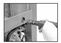
▶ Drill out the inner tank wall behind according to the required connection diameter.
