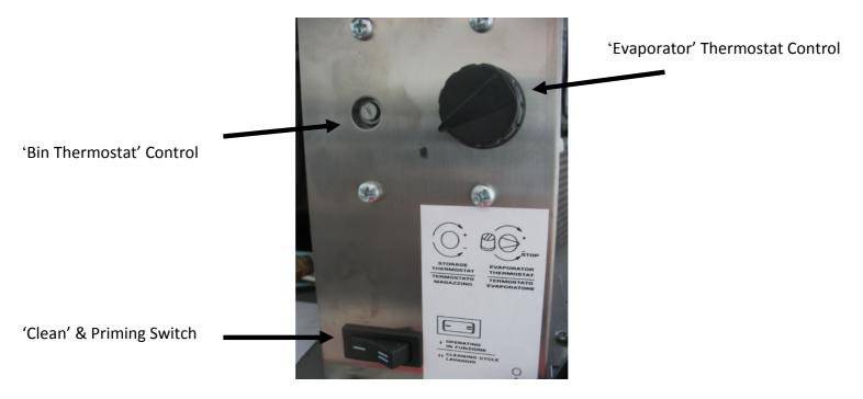
NOTE – During install/commissioning, adjust the 'Bin Stat' control fully clockwise to prevent nuisance tripping off under a bin full condition...
