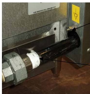
PHOTOGRAPH 20. EQUIPOTENTIAL AND GAS INLET CONNECTION.
