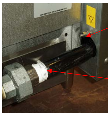
PHOTOGRAPH 20. EQUIPOTENTIAL AND GAS INLET CONNECTION.
