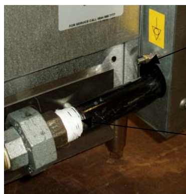
PHOTOGRAPH 20. EQUIPOTENTIAL AND GAS INLET CONNECTION.
