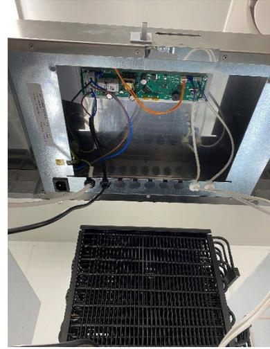
Once whatever work required have been performed, the controller box lid is re-fitted using the two torx 25 screws and the top panel is re-positioned and fixed by use of the M5 screw. Once the top panel is positioned and fixed correctly, the top panel will be placed like shown on the below picture (seen from the compressor compartment)
