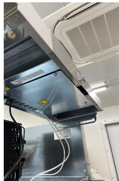
On the back of the top panel there is a rather large lid, which can be dismantled by removing the two torx 25 screws holding it. Once the lid has been removed there is direct access to the above-mentioned parts and connections.
