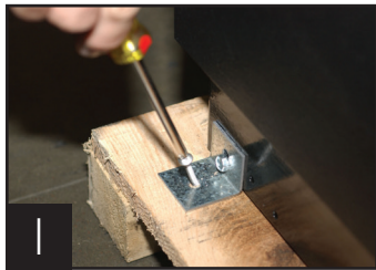
1 Removing bracket from skid.
