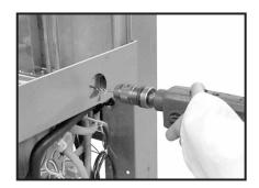
▶ Drill out the inner tank wall behind according to the required connection diameter.
